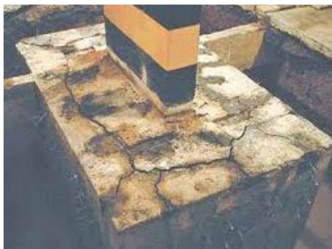
Figure 5. Pile cap block with cracked upper surface, with openings in the order of 25mm [37].
