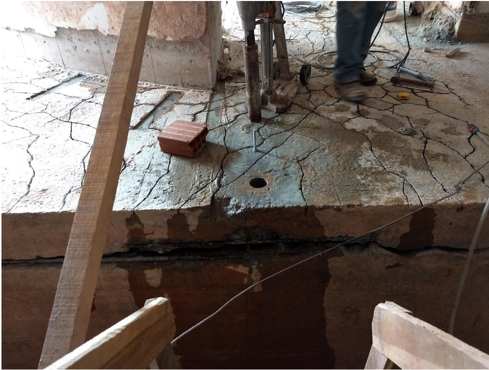
Figure 27. Cracking in pile cap and place where a sample was extracted.
