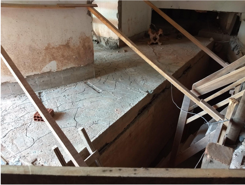
Figure 25. Horizontal and map cracking in pile cap block.
