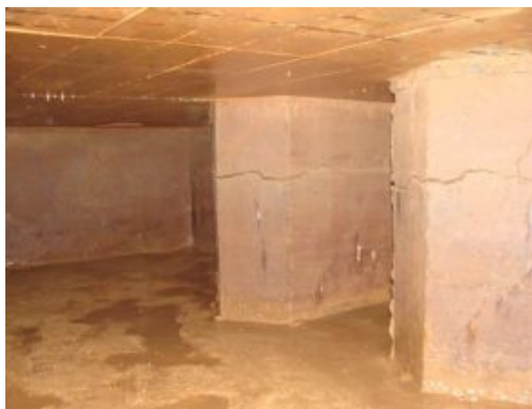
Figure 2. Pile cap foundation with longitudinal cracking [11].
