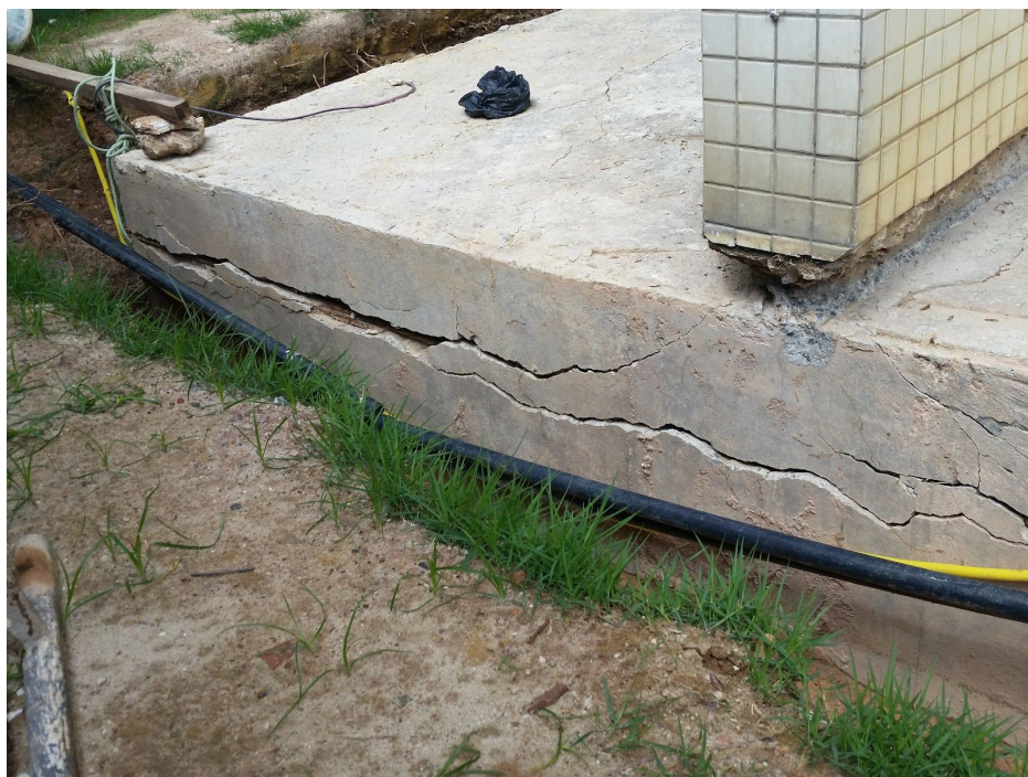
Figure 30. Longitudinal cracking with a large opening in the pile cap block S(P6+P9) [11].
