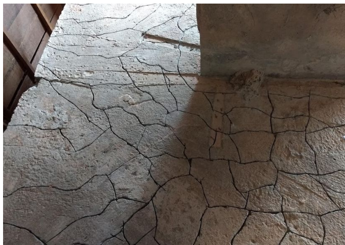
Figure 49. Map cracking on the surface of the pile cap block.
