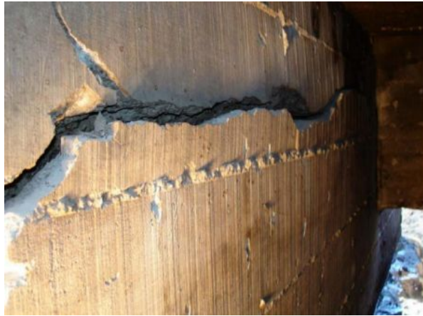
Figure 3. Longitudinal crack and relative horizontal displacement [25].
