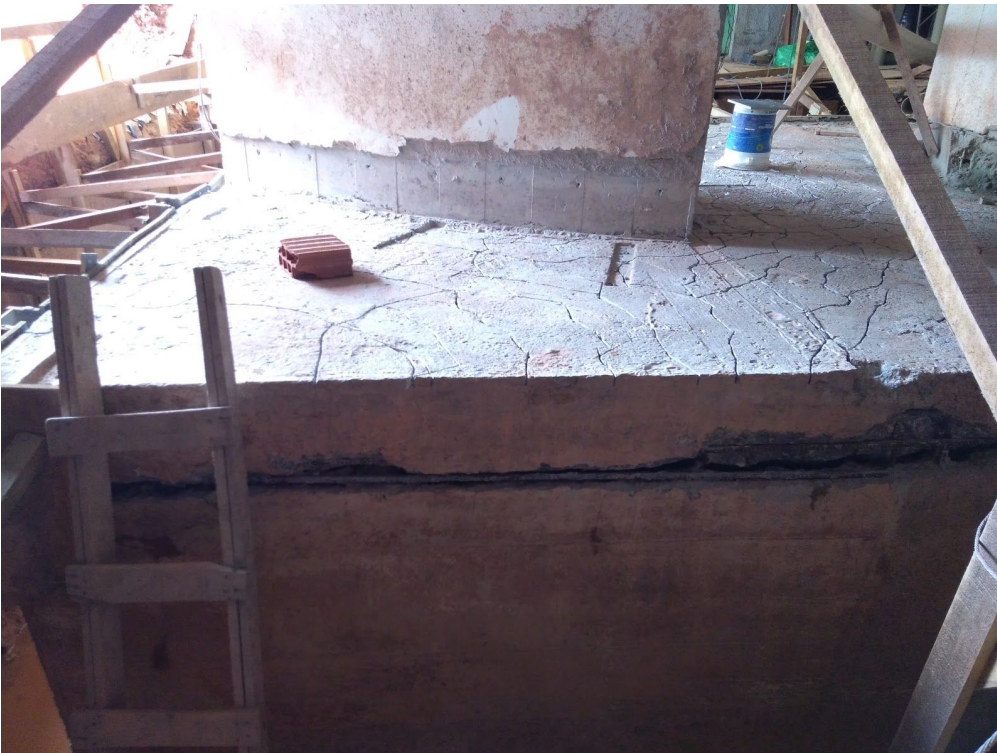
Figure 26. Horizontal and map cracking in pile cap block.
