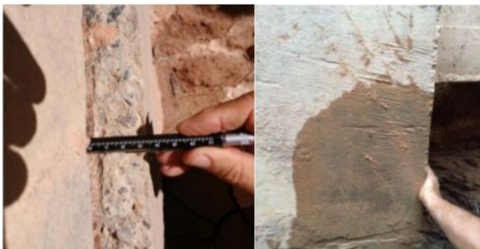
Figure 32. Horizontal displacement and sloping cracks [11].
