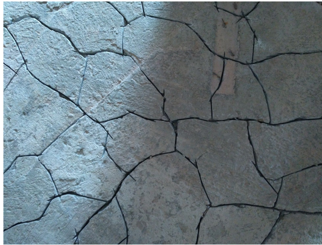
Figure 29. Cracking in map format on the surface of the pile cap foundation S(P1+P8+P32).
