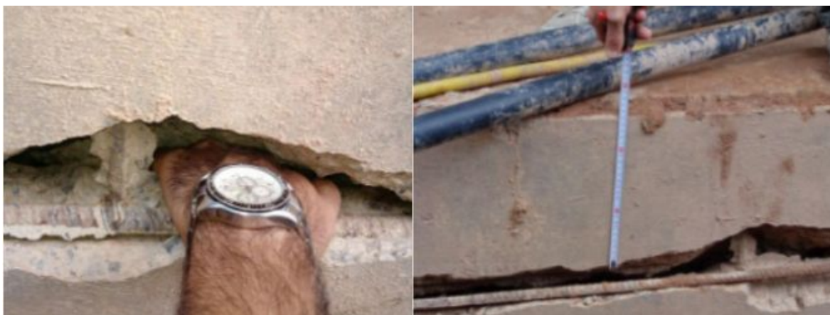
Figure 31. Opening of cracks and depth of the crack [11].
