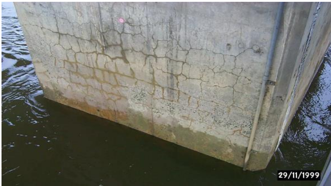
Figure 17: Pier 6 of the Bellevue Bridge with map cracking in the tidal zone (DEF). (Godart and Divet, 2013)
