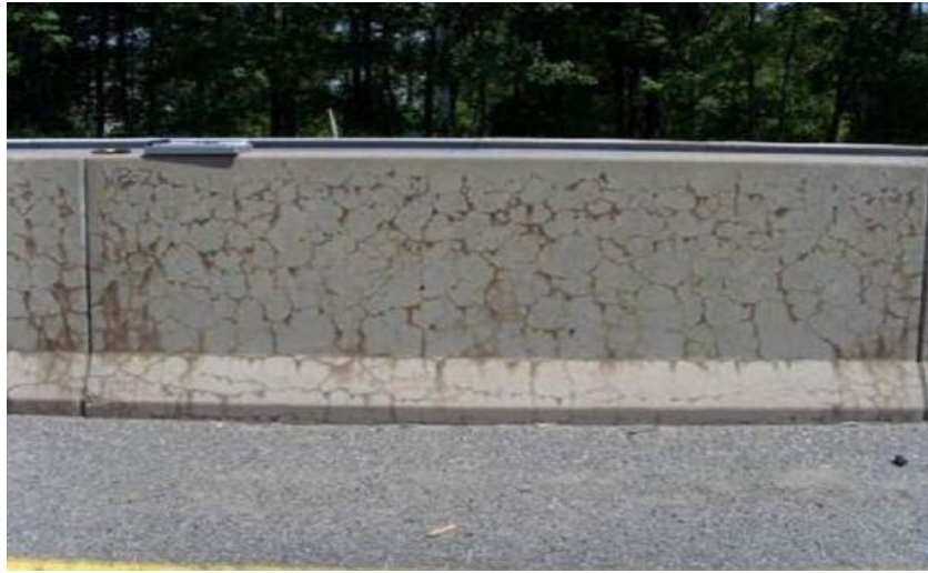
Figure 16: ASR damage on barrier walls. (Thomas et al, 2013)
