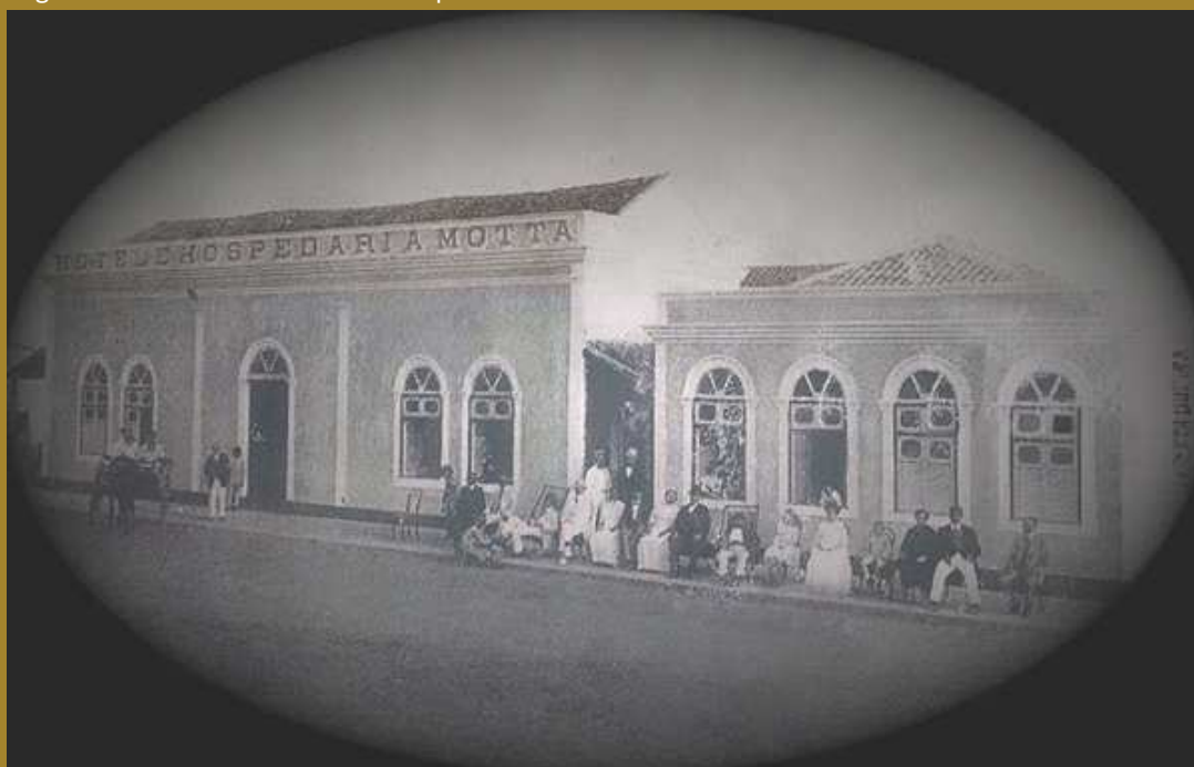
Figura 14 – Fachada do Hotel e Hospedaria Motta - Garanhuns-PE
