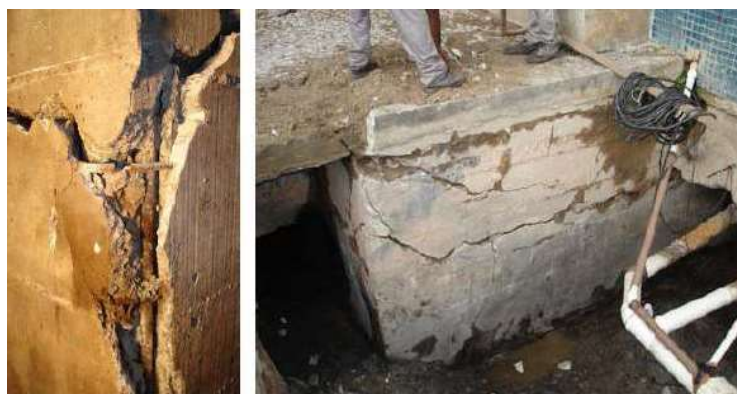
Figure 2.2. Crackings caused by AAR on the foundation blocks (pile caps) of a public building with 13 floors (adapted from ANDRADE et al., 2006a).
