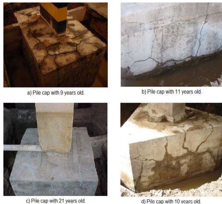
Figure 2.3. Crackings caused by AAR on buildings at the RMR (adapted from ANDRADE, 2006).
