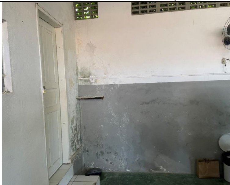
Quadro 70- Parede externa a Copa 2
